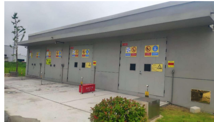
Hazardous Waste Warehouse (Sieyuan Toshiba)
