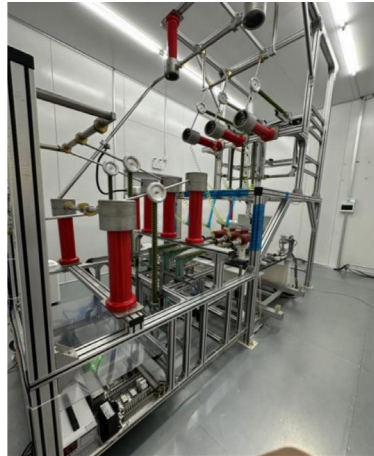
Automated Test Station
