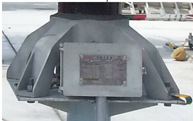
EN/Fig. 8.3 Connection between Product and Foundation
