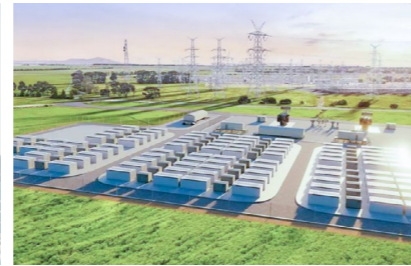
Standalone Energy Storage Stations
